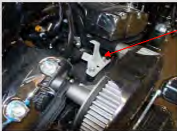
New ACR Bracket to hold wires
