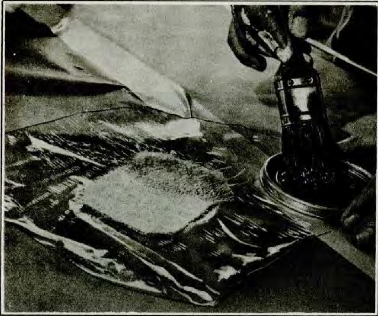
Figure 2J-10. Applying Resin to Mat
